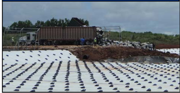
Layon Landfill—Guam Solid Waste Authority
