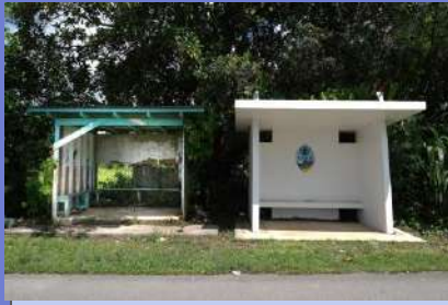
School Bus stops repaired by DPW Building Maintenance
